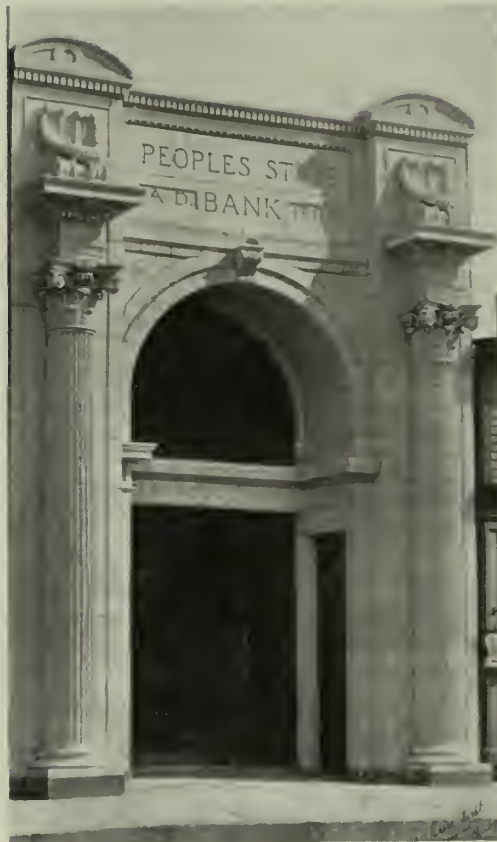
PEOPLES STATE BANK, CROWN POINT, IND. Built of full glaze cream terra cotta made by the Northwestern Terra Cotta Company. Beers & Beers, Architects.
